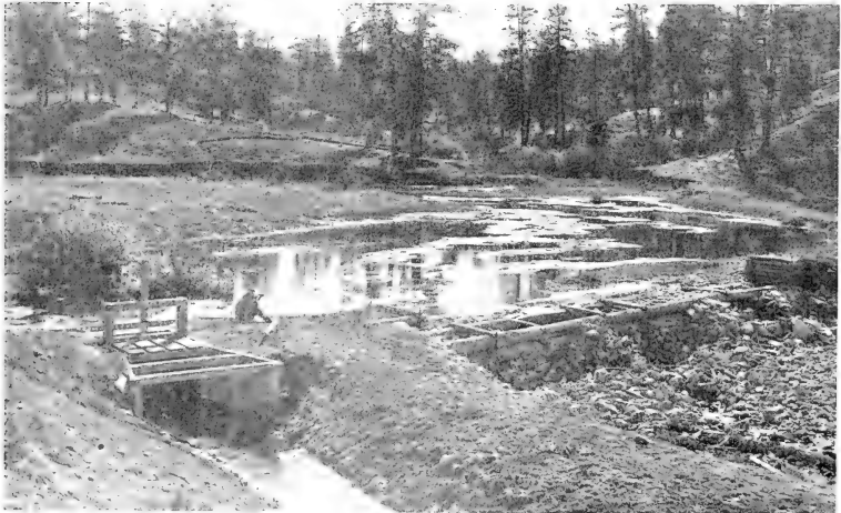
HEADWORKS OF WHEATFIELDS CREEK DITCH, BUILT BY NAVAJOS UNDER GOVERNMENT SUPERVISION.
